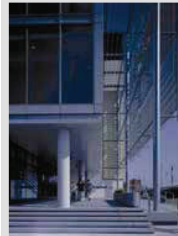
Loxley House (offices) in Nottingham.
