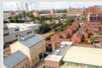
Barkantine Estate, London: retrofit community energy network using Combined Heat and Power (CHP) to service over 700 dwellings, a leisure centre/swimming pool and primary school.
