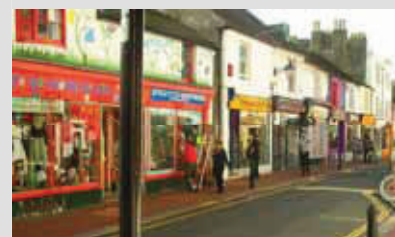
Upgrading of existing buildings: Sydney St
