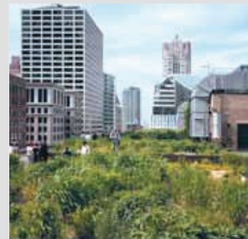
Chicago City Hall: green roof (picture: Mathew Frith)
